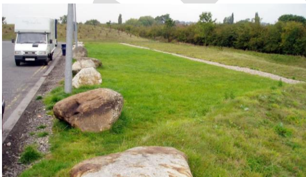
Figure 3. 9 Example of filter strips (Source: Susdrain)
