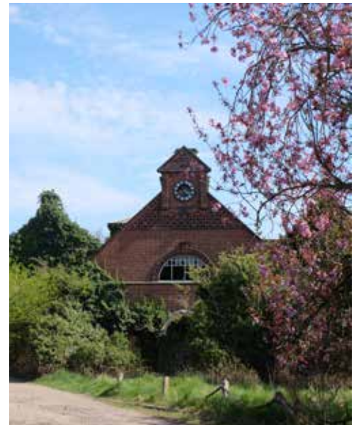
Top: The listed former Trowse Railway Station building Bottom: Former pumping station building, east of the railway line
