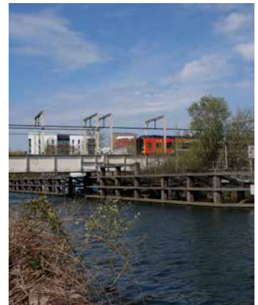
Top: Existing railway underpass Bottom: Existing Trowse Rail Bridge
