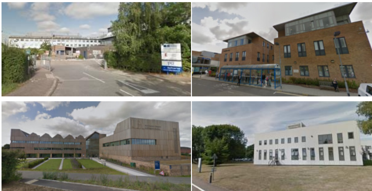
Figure 21: Norwich Research Park Site Photos
