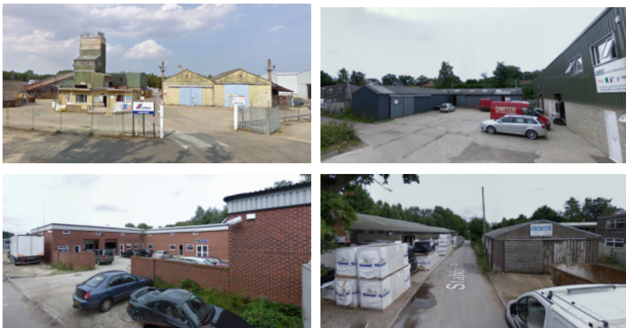
Figure 14: Lenwade Industrial Estate Site Photos
