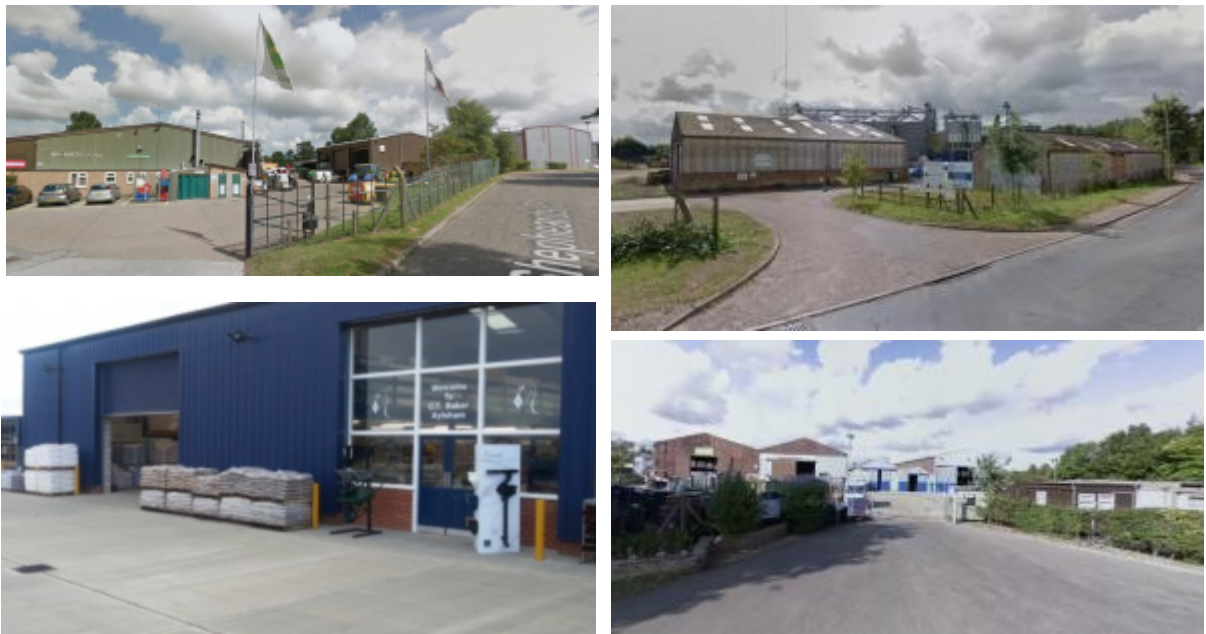
Figure 6: Dunkirk Industrial Estate Site Photos
