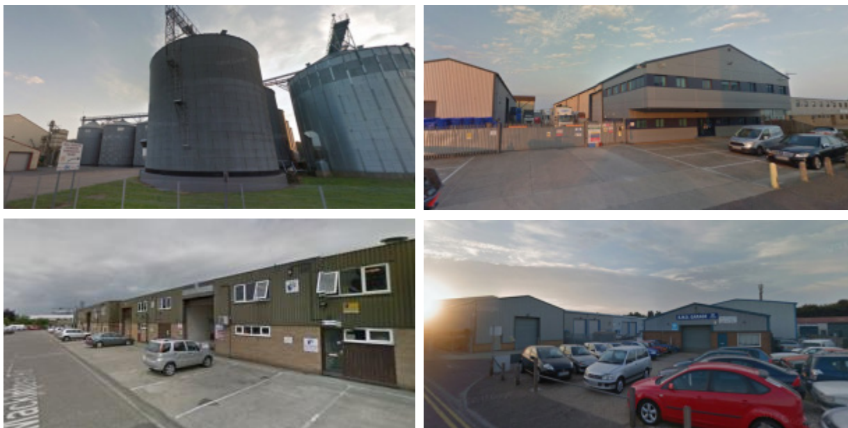
Figure 17: Rackheath Industrial Estate Site Photos
