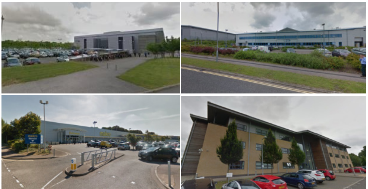
Figure 19: Broadland Business Park Site Photos
