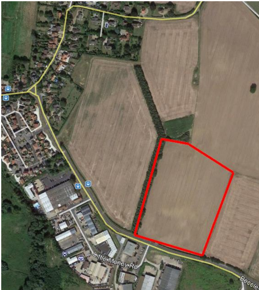
Fig. 3 – Aerial image illustrating the position of our client’s site in respect of established residential properties, employment and the Loddon development boundary. Source: Google Earth
